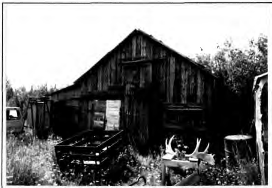
Figure 24. The Miscovich House/Uotila Shop, 1993. The view is looking southwest.
